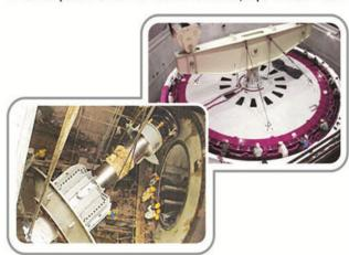
Complete Electro Mechanical work including assembly and installation of bulb nose turbines (8 x 23.7 MW), generators, draft tube gates, intake gates and Hydro Electric Equipment for 184 MW Chashma Hydro Power Project EPC contractors Marubani Corporation/ Fuji Electric. in 2002
